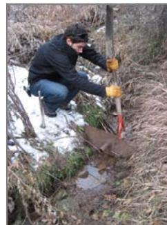
Engineer Brendon Langenhuizen installs a stream gage below Juárez Spring.
