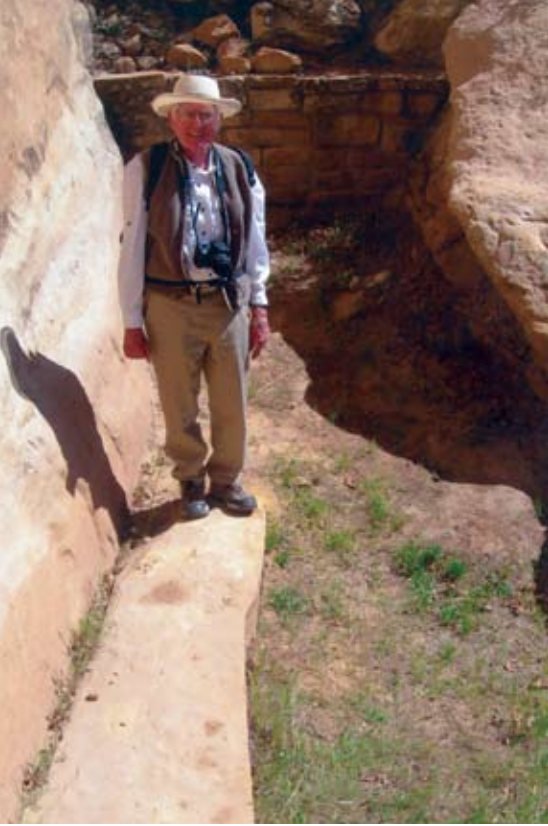
Figure 9. The author stands in the Mug House Cistern, which collected water from a drainage notch 85 feet above. Its capacity is 4,000 gallons.
