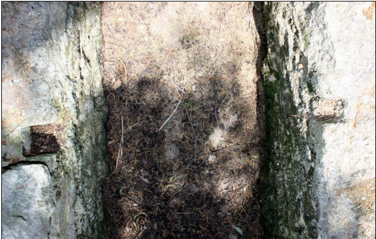
Figure 7. Notches for slide gate.
