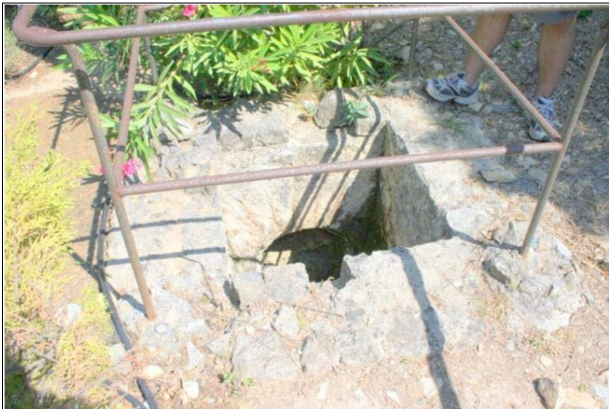
Figure 3. Regard coin rues shaft and top of tunneled section.
