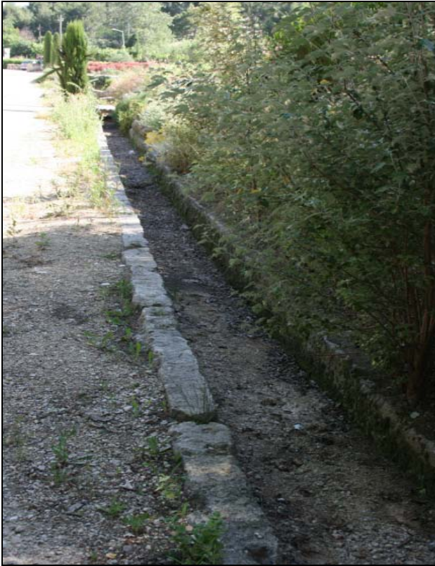
Figure 5. South aqueduct la burlande channel – downstream of basin.
